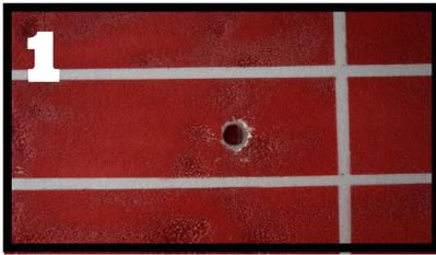
Drill for 2 seconds into external brick wall to create counter-sunk indentation
